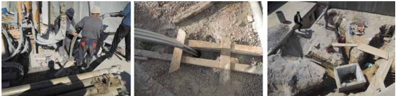
Figure 15. Borehole drilling and assembly of geothermal probes
