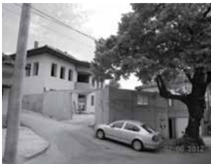
Figure 10. First phase of works at the Vrbanjuša House (2012.)
